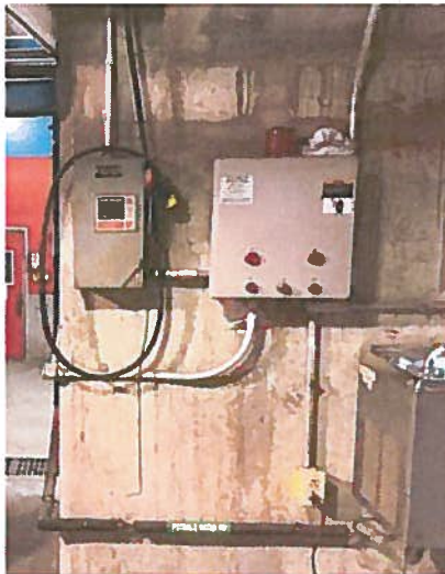
Gland Seal Leak Off Pump 1 Standard
