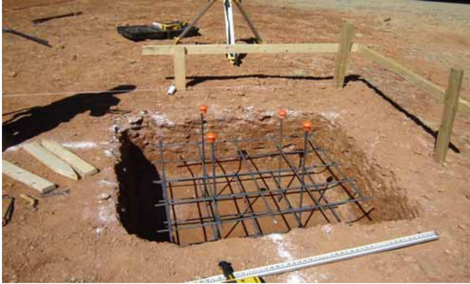
View of excavated corner footing with rebar installed
