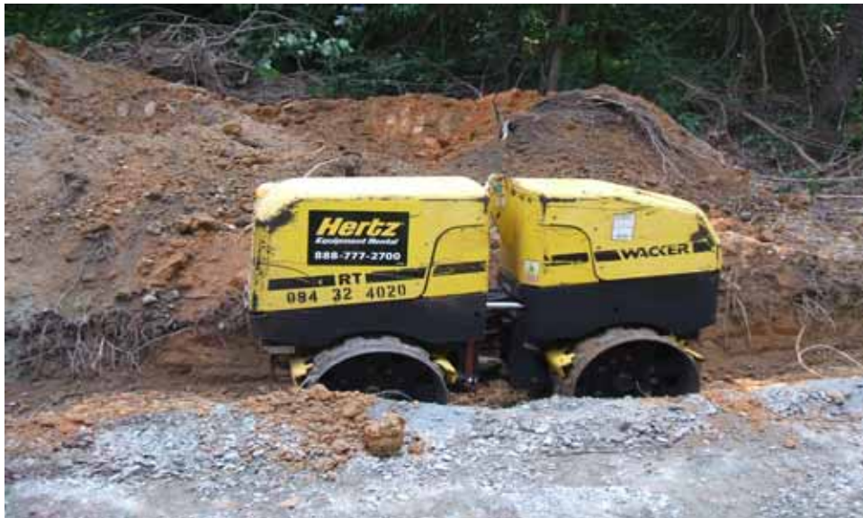
View of trench compaction adjacent to DRW-2
