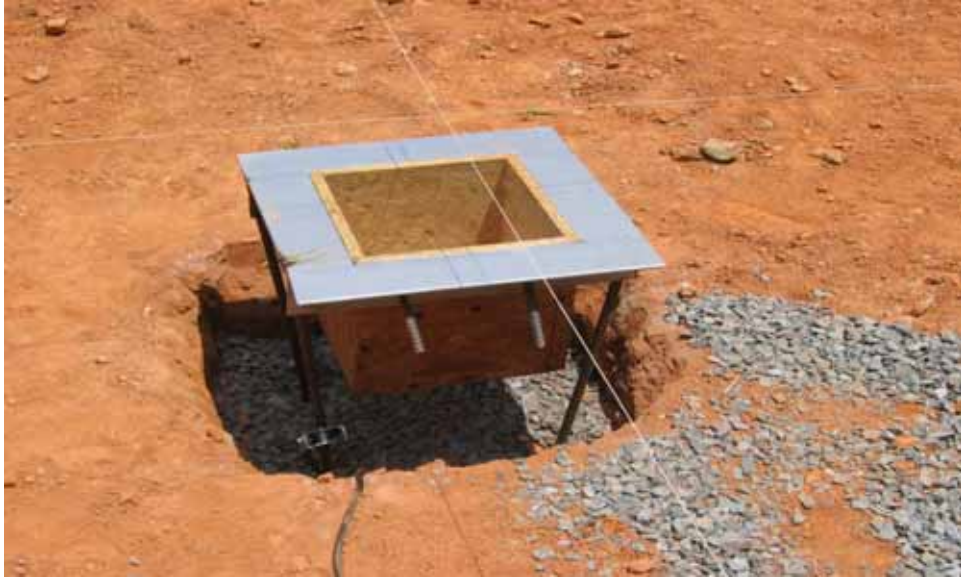
View of sump in center of future slab in equipment room
