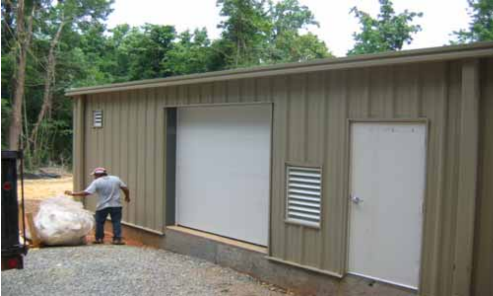
View of completed exterior of building
