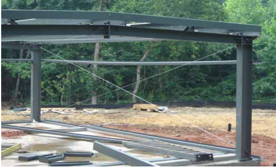
View of structural steel installation
