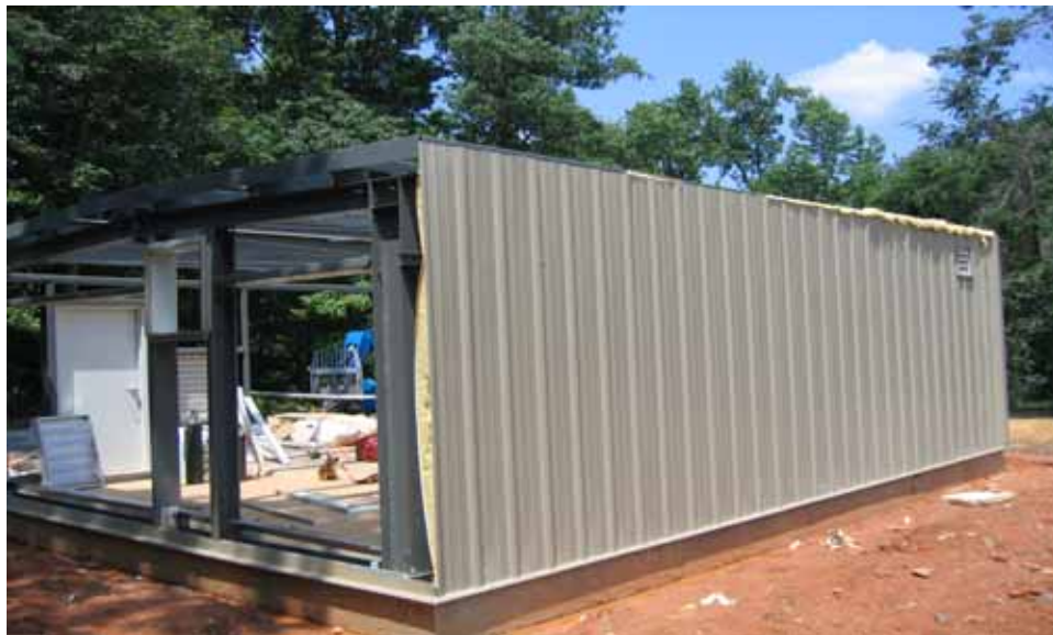
View of exterior siding installation
