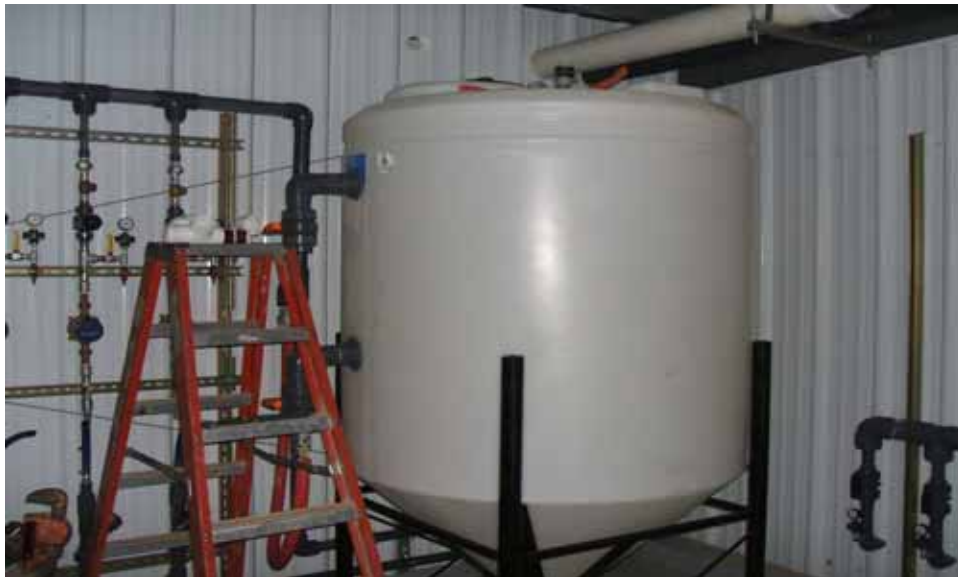
View of building interior and settling tank
