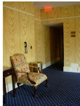
Graham Memorial Hall Area of Rescue Assistance (upstairs) provides a telephone that calls the downstairs Fire Alarm Panel to speak with Fire Department.
