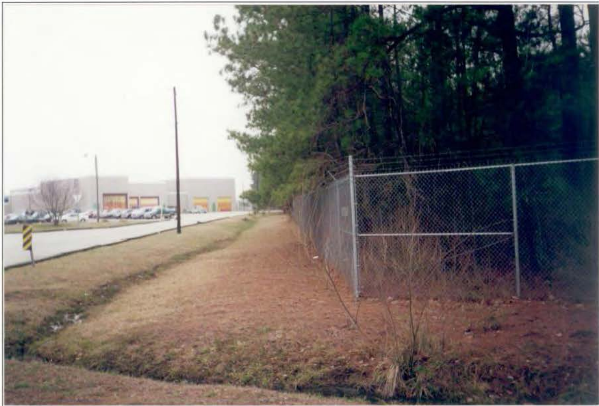
View of disposal area facing southwest.
