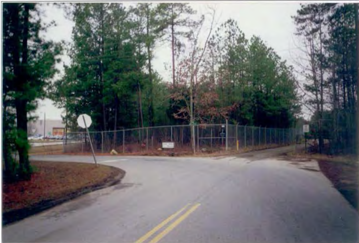
View of disposal area facing southwest.
