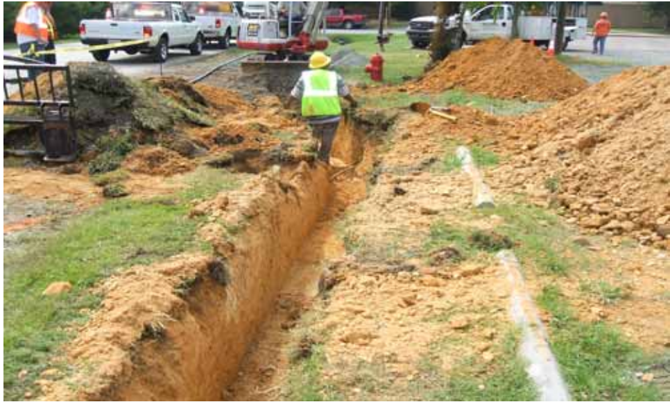
View of installation of discharge line to OWASA manhole
