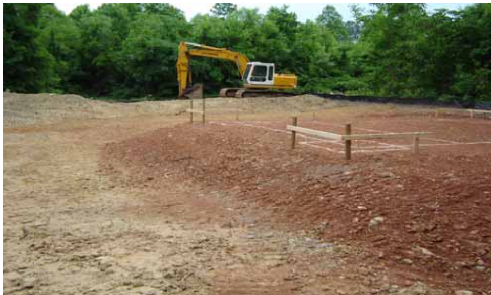
View of building pad following site clearing and soil replacement
