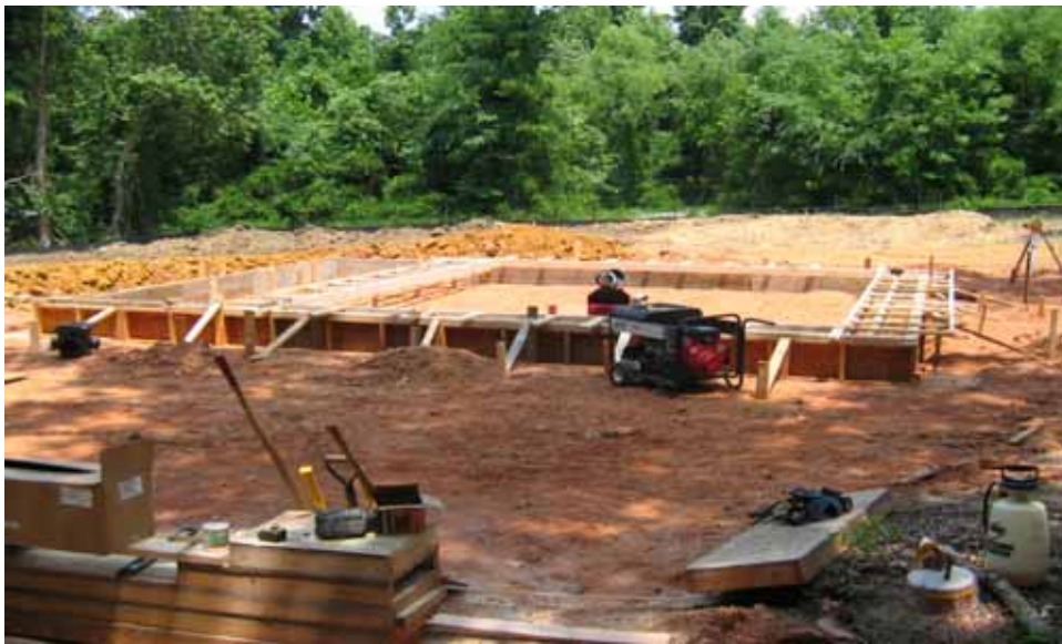
View of forms for concrete pad. Left side of pad is future equipment control room. Right side of pad will contain groundwater treatment equipment
