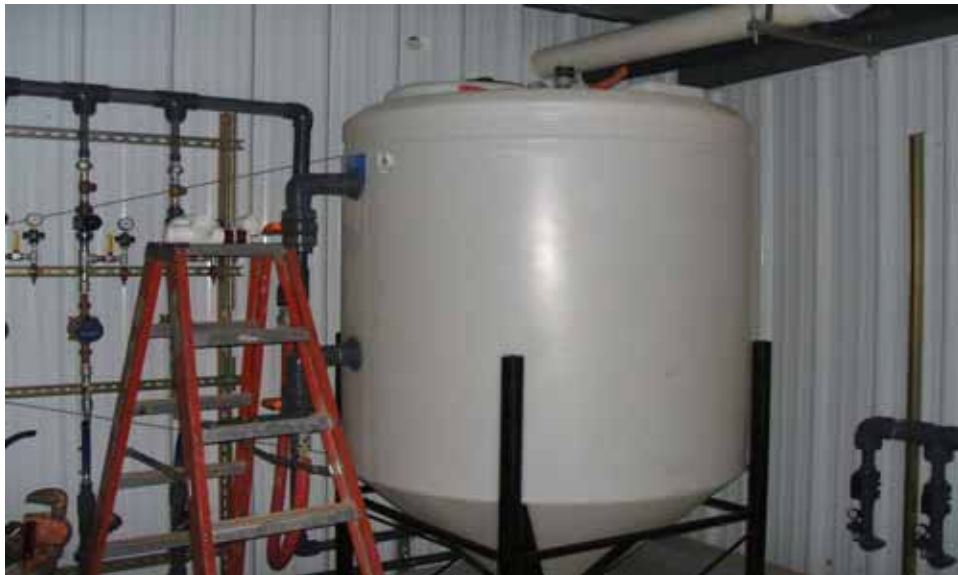
View of building interior and settling tank
