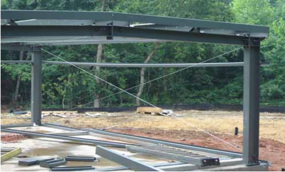
View of structural steel installation
