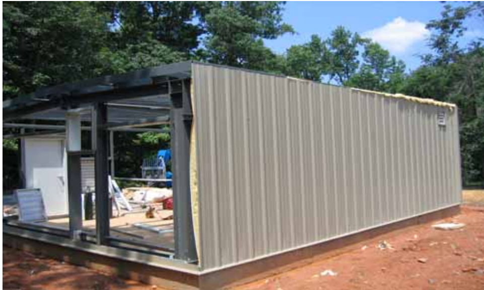
View of exterior siding installation
