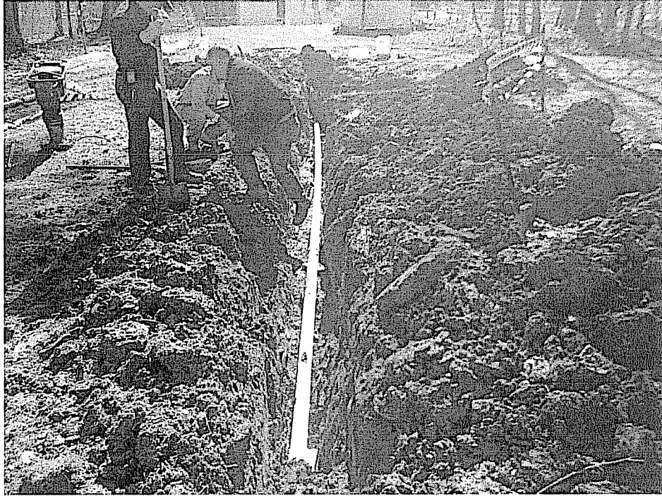
Picture 3 – Open trench and new piping prior to backfilling.
