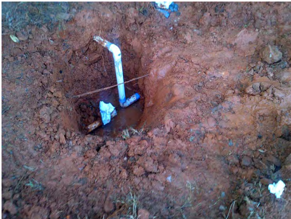
Picture 2 – Repair completed.
