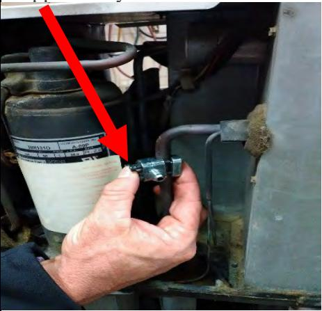
The gauges should be turned off and then connected to the high and low sides of the unit to be recovered from. Red goes to the high side; Blue goes to the low side.
